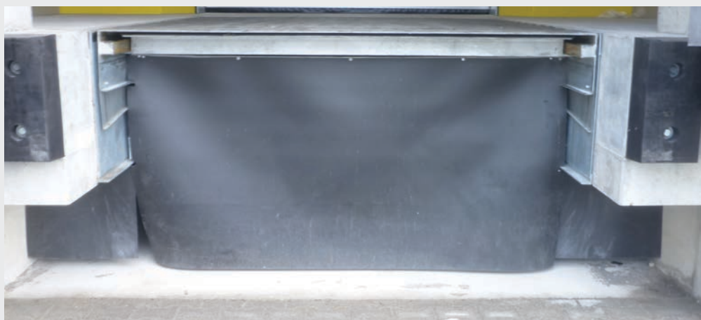
Cover curtain for tail lift recess
